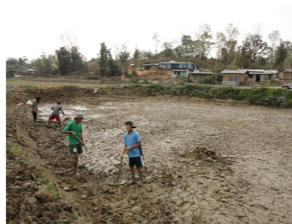
Fig: Renovation of old pond
