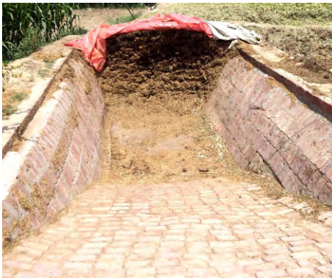
Pakka Trench Silo Pit
