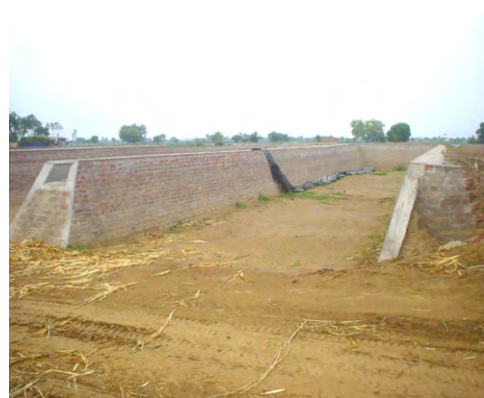
Pakka Bunker Silo
