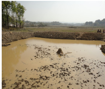
Fig: A view of construction of new pond
