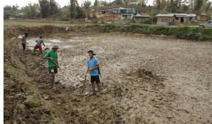
Fig: Renovation of old pond
