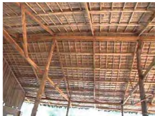
Traditional wood, bamboo and thatch roofs
