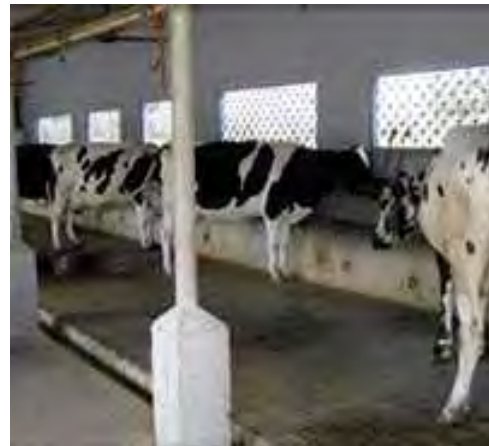
Grooved concrete flooring under covered area of shed for housing of cattle
