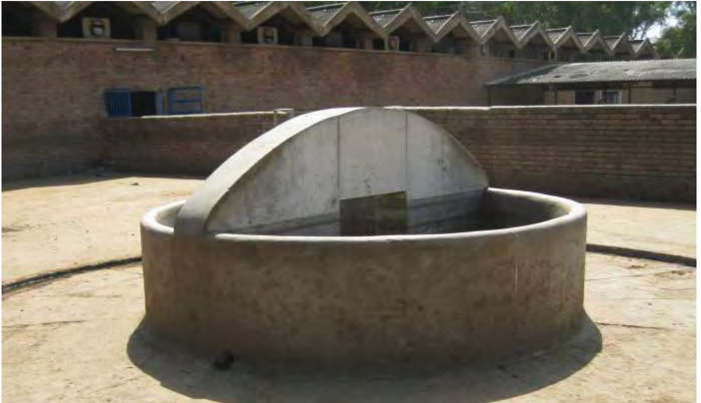
Water trough with round edges to prevent injury to the animals
