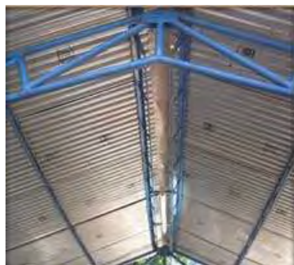
Corrugated aluminium sheet roofing in cow
