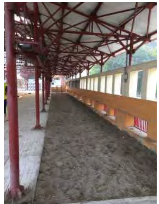
Lame animal sheds should have a provision of sand bedded floor for the comfort of animals
