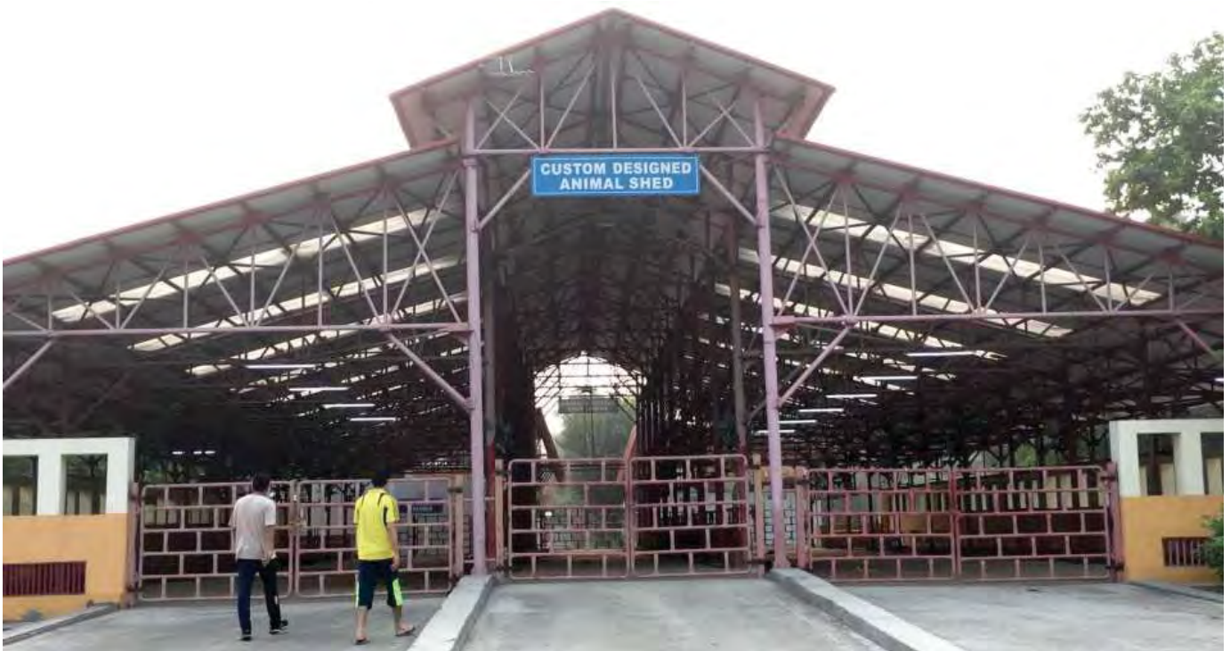
Distant view of 3 hinged gates in the modern head to head cattle sheds (2 in to the entrance of cattle sheds and 1 in to the central feeding passage)
