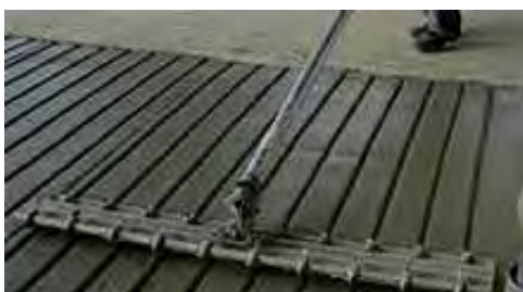
Grooved concrete floor under construction
