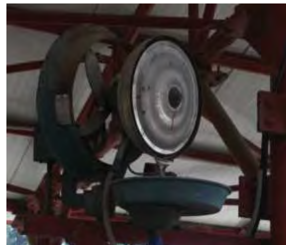
Picture of a fan fitted with fogger for keeping the temperature inside the shed low
