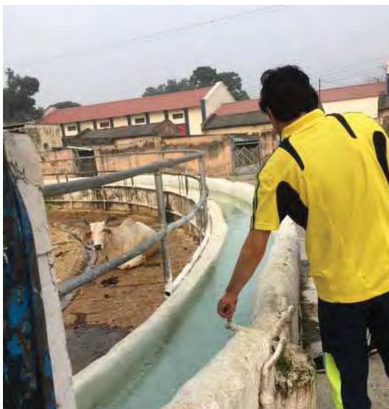
Water trough at the corner of a shed with a tap and fence over it to prevent animals jumping into the trough
