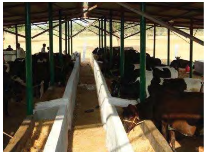
Buildings should be placed and constructed such that direct sunlight can reach the platforms, gutters and mangers in the cattle
