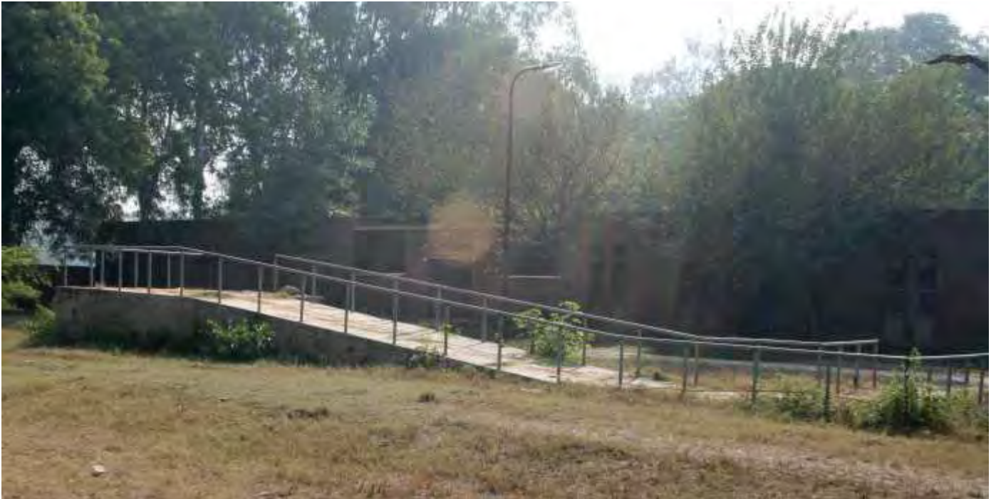
Permanent ramp made of concrete for loading and unloading of animals.
