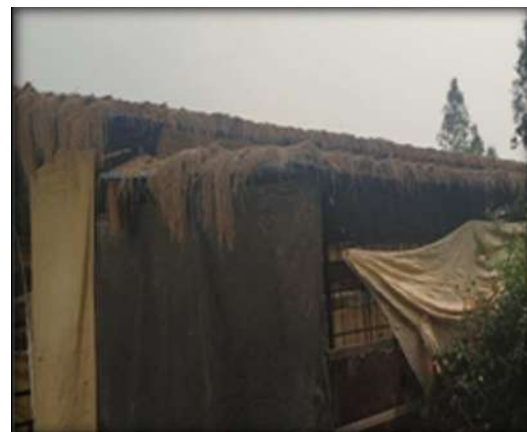
Poultry house roof and thatching material
