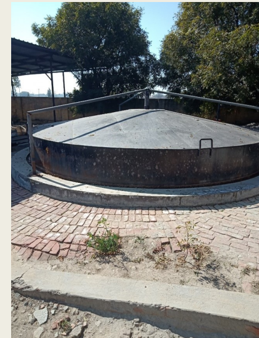
Picture-8: Biogas generation for handling of dung generated from Dairy Farm
