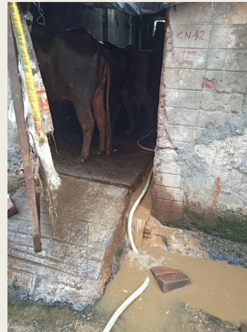
Picture-3: Floor Cleaning Wastewater discharged in drain from Shahbad Dairy Farm
