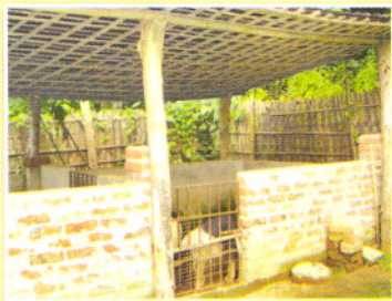
Brick floor, pucca walls with bamboo roof -better housing under rural condition
