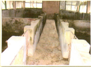
Concrete floor, pucca walls with asbestos roof
