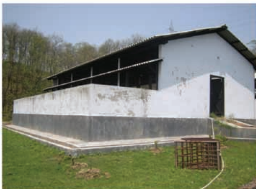
Fig 5: A concrete pig sty (gable type)
