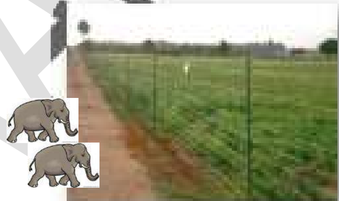
Erected by Karnataka FD
